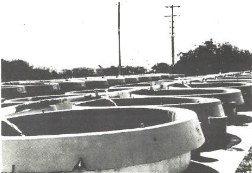
Plate 4. Small tanks used for research and medication purposes in Area 8.
