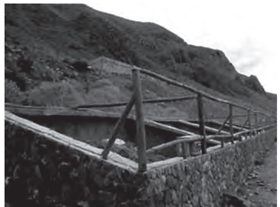
Figure 4. Almost finished units, Gran Canaria.
