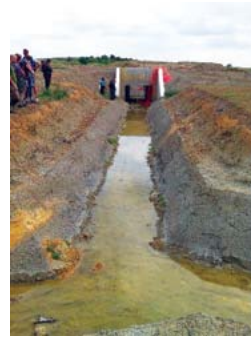
Figure 5. New tunnel at Hampton Nature Reserve, Peterborough, UK.
