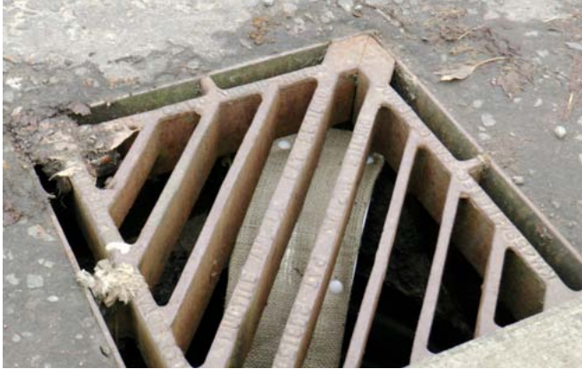
Figure 3. Ladder installed within a gullypot. Photo credit: Rose, T.
