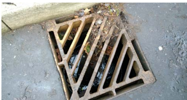
Figure 7. Leaf litter and debris build-up at the ladder top, which facilitates easier escape through the grating. Photo credit: Rose, T.
