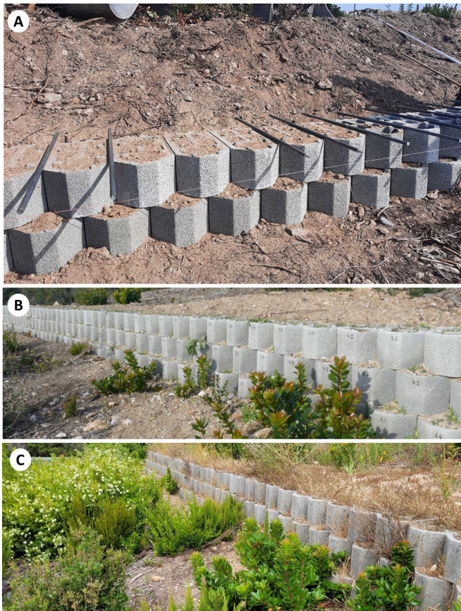
Figure 1. Views of an experimental breeze block wall constructed on an excavated surface with the breeze blocks set apart to give standardised crevices between them, in which Euleptes europaea and young Hemidactylus turcicus could take refuge, as photographed in - A. September 2022, B. January 2023, C. June 2023
